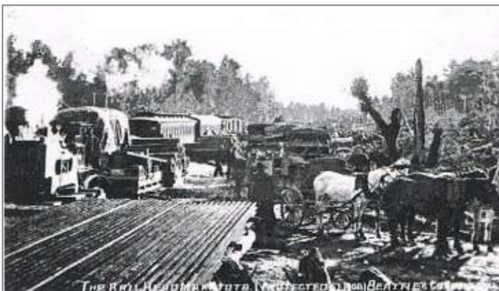
PROTECTED 1. 7. 1908 By now, the railheads were not far apart. Near Makatote, a large viaduct was built for the railway. Construction took two years and was completed around the end of 1908. This view shows a recently arrived train in the background, with a coach waiting to take the passengers on to the other railhead.
